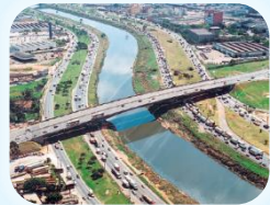
Beginning of the Tietê River Depolluting Program
