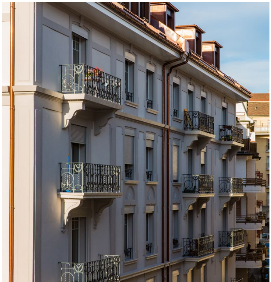
Comprehensive renovation on Rue des Echelettes in Lausanne
