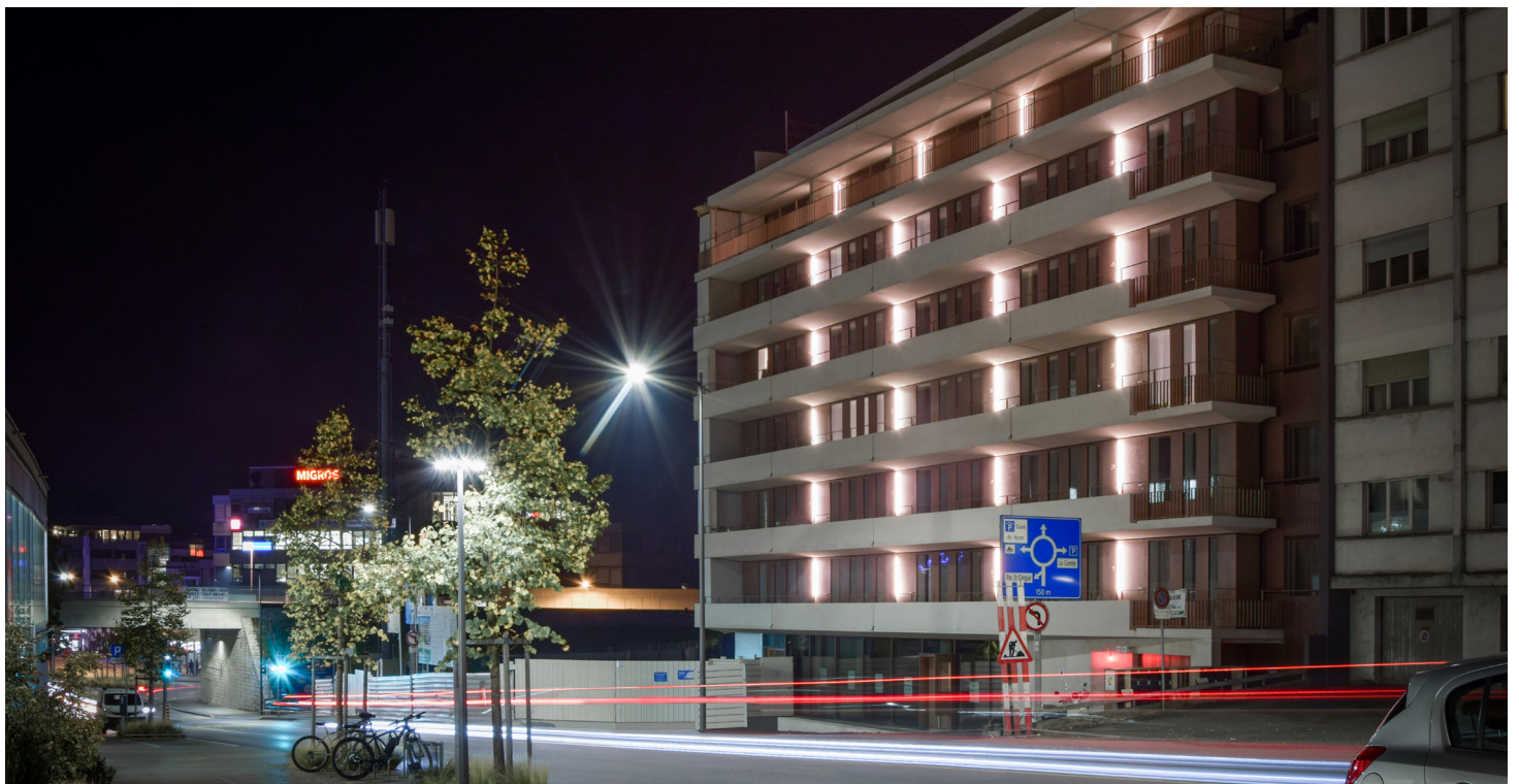
New building on the Rue de la Morâche in Nyon (VD)
