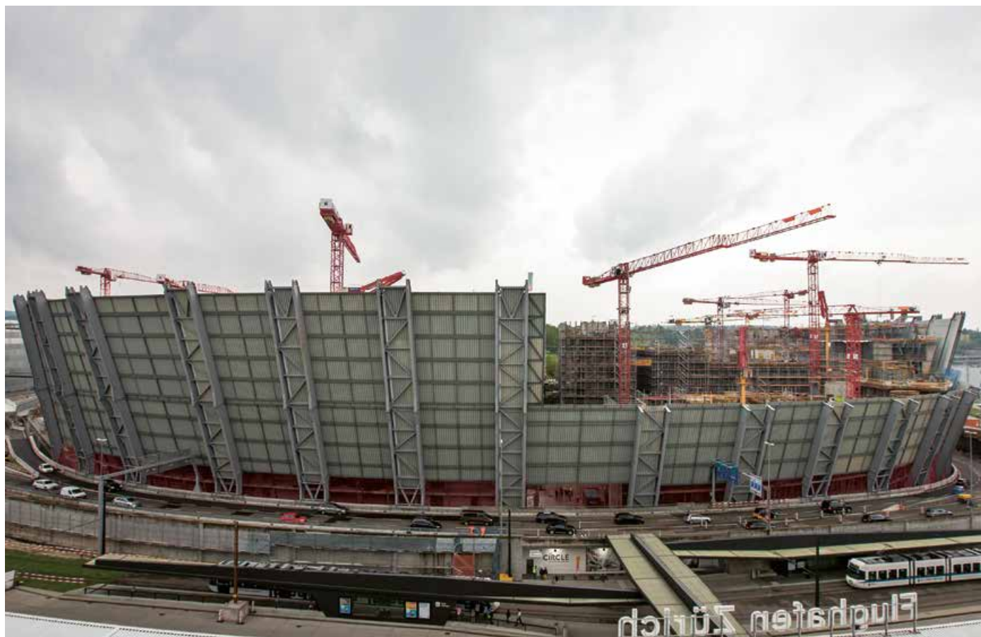
"The Circle" construction site at Zurich Airport | Keystone/Alexandra Wey
