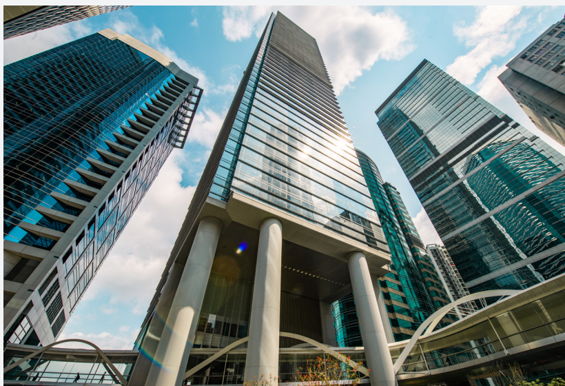
One Taikoo Place, Hong Kong An award-winning triple Platinum grade certified (LEED, BEAM Plus and WELL) green and healthy building. >
