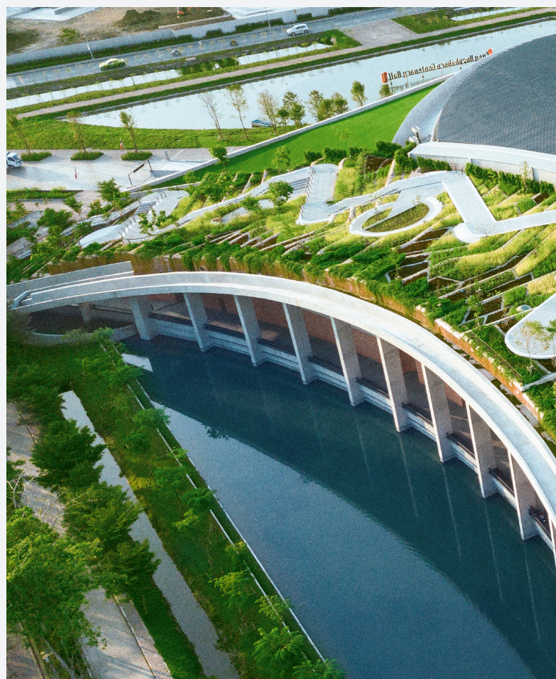
Thammasat University Rooftop Farm (TURF) Asia's largest rooftop farm, built with Firestone's UltraPly TPO 1.5mm – 20,000m 2 green roof in Thailand. >
