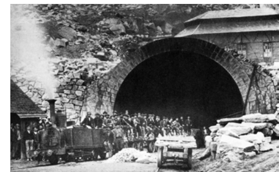
Construction of the Gotthard tunnel, 1880
