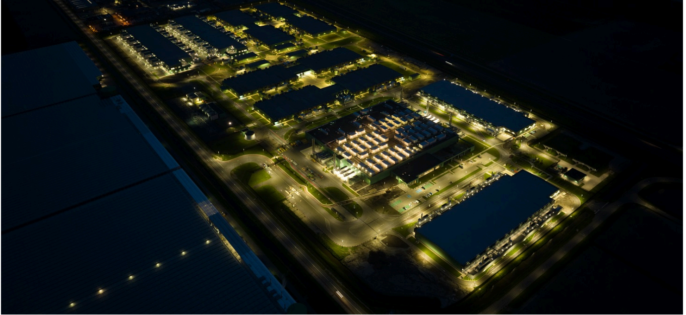
A large-scale data center in the Netherlands (Shutterstock)
